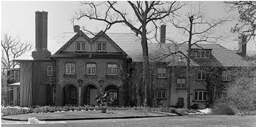
The front façade of the George Pick House, Highland Park, 1970s. The present ceiling light can faintly be
